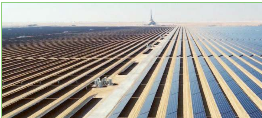
Mohammed bin Rashid Al Maktoum Solar Park II
