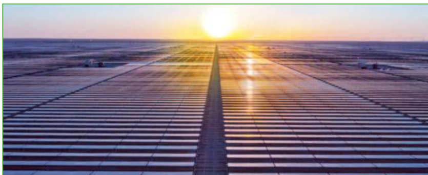
Sakaka Photovoltaic Solar Project
